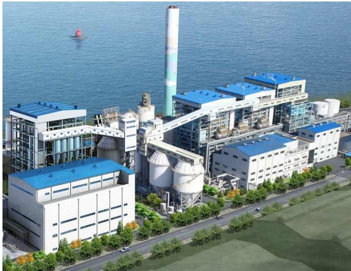
Biomass Combined Heat and Power (CHP) Station With a consumption of 40,000 tonnes wood or other biomass, a 1 MW class combined heat and power (CHP) station generates around 20 million kilowatt-hours electricity and 50 million kilowatt-hours heat annually. In principle, such a power station functions like a coal-fired power station.
